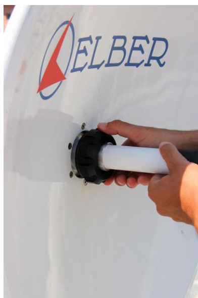
Figure 6: Feeder installation
